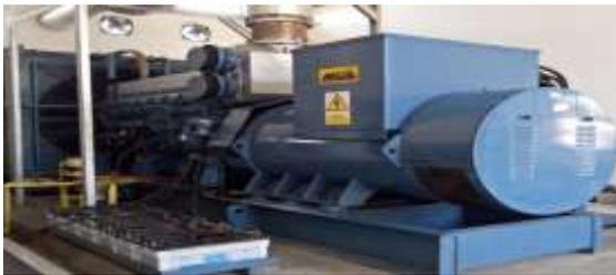
Gambar. 2 Mesin Diesel Mitsubishi 2000 kVA
